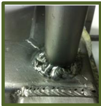
Figure 11. Poor sanitary welds are not cleanable at a microbiological level
