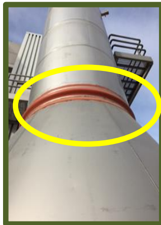
Figure 17. Example of an exterior expansion joint that needs regular inspections
