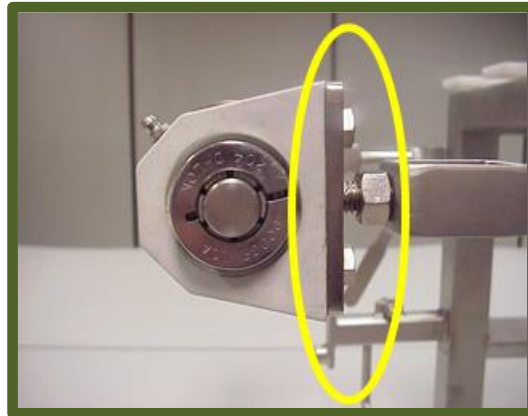
Figure 37. Sandwich area formed by the bearing housing and framework where Listeria spp. had established a niche and the framework had rusted.
