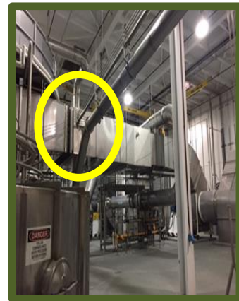
Figure 18. Example of an interior expansion joint that needs regular inspections
