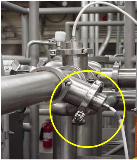
Fig. 23. Accumulation/niche created by reassembling the probe facing down instead of up
