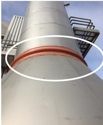
Fig. 17. Example of an exterior expansion joint that needs regular inspections
