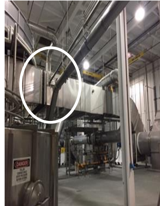
Fig. 18. Example of an interior expansion joint that needs regular inspections
